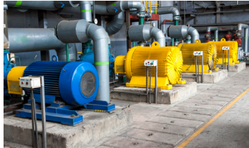
Plant / Equipment Installation
